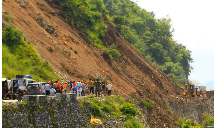
Figure 5. Landslide in hilly terrain
