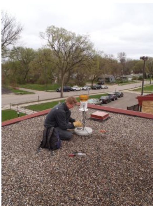
Figure 3. An automated rain gauge station on the Roof of Thomas Edison High School Gymnasium building, Minneapolis, Minnesota.
