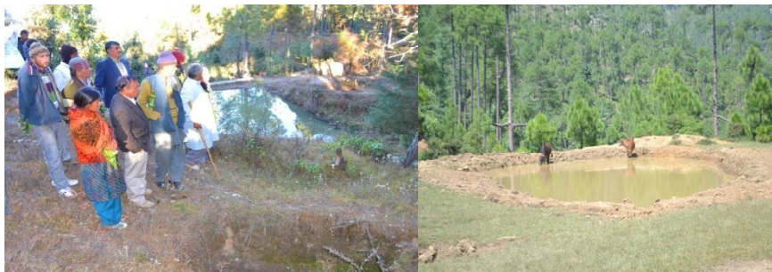
Construction of percolation tank at lower slope for water recharging
