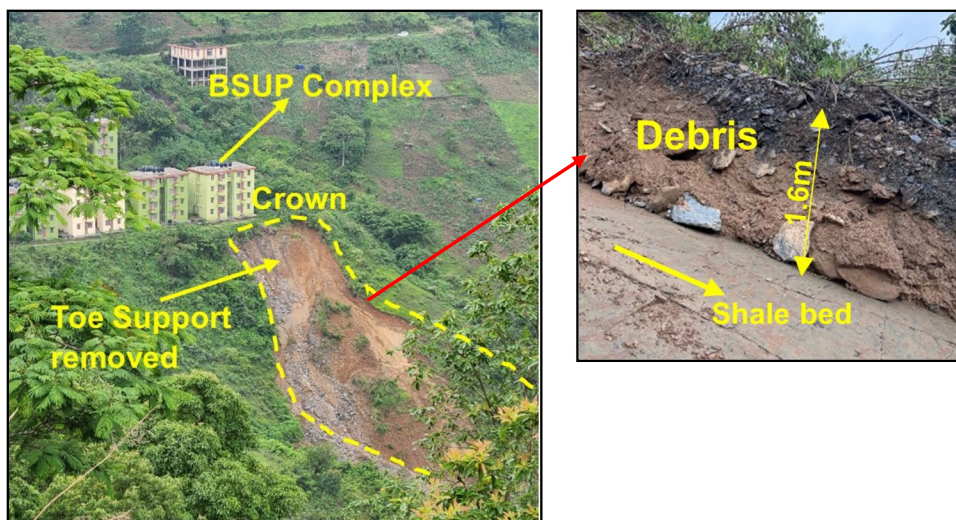
Fig. 9 Landslide in BSUP complex, Durtlang, Aizawl. The yellow line indicates the boundary of the landslide and the overburden material above the shale bed (1.6 m thick)
