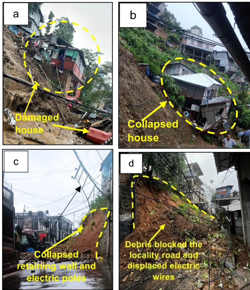
Fig. 3 Random pictures of landslide damages in and around Aizawl. a, b Damage and displacement of houses caused by debris flow. c, d Road blocked and displacements of electric poles and wires due to collapse retaining wall
