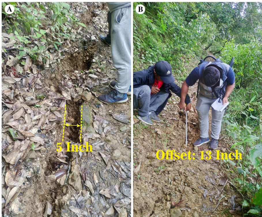
Fig. 6 Picture showing different scale of fractures occurred during the Champhai Earthquake: a 5-inch crack observed in Samthang village, in the epicentral zone; b offset of 13 inches recorded from Chawngtui village
